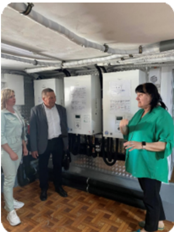
Controllers of the Heat Pumps in the basement
